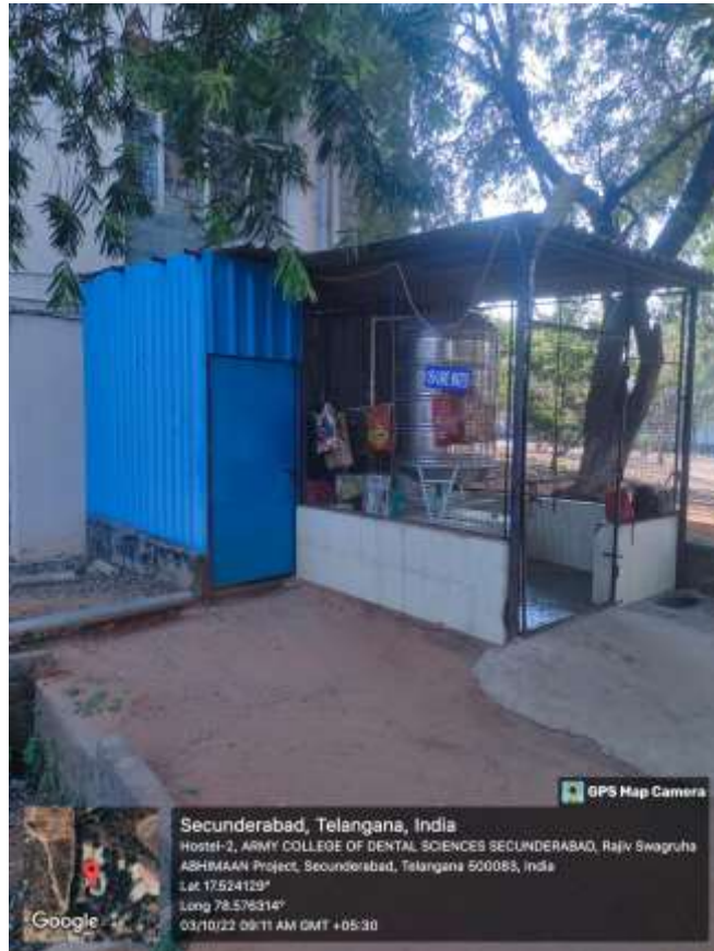
Fig-24: Save water signages
