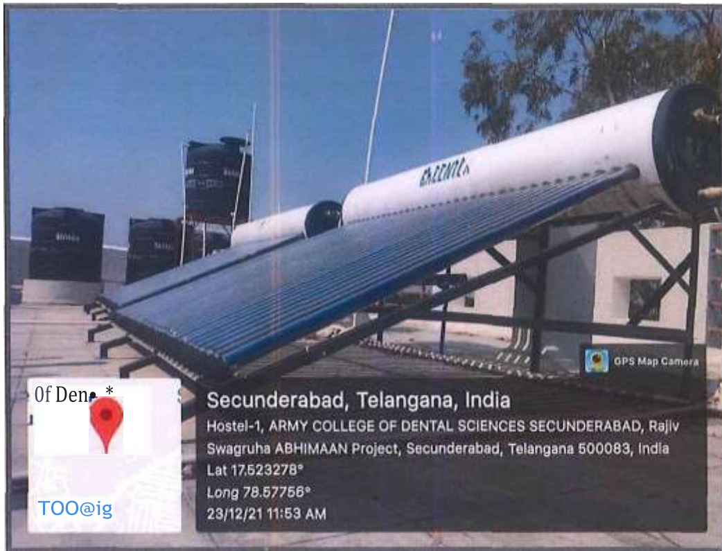
Fig-12: Water tank in girl's hostel
