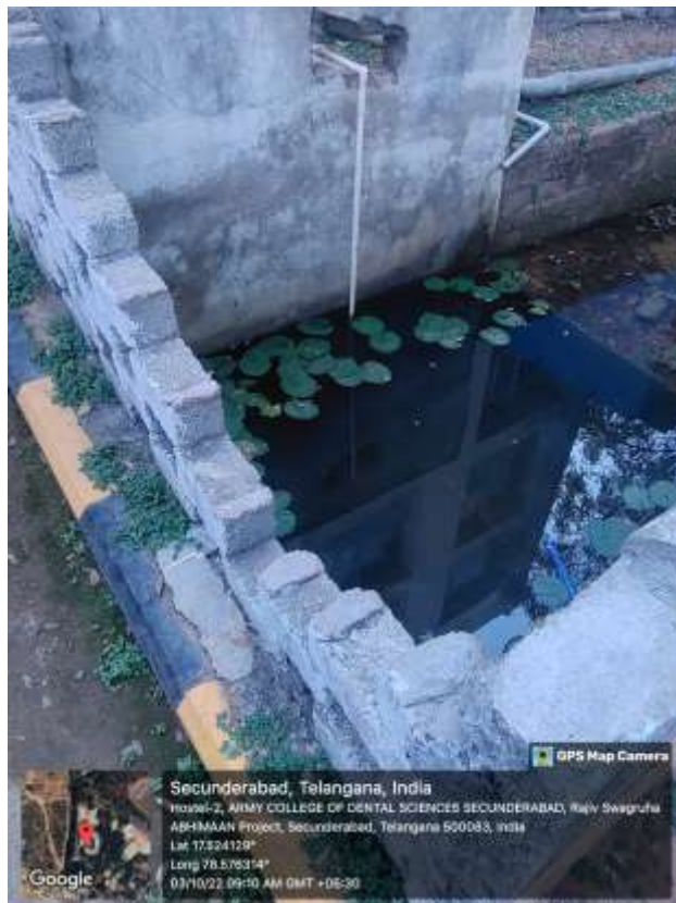
Fig-9: Water tank in the college premises
