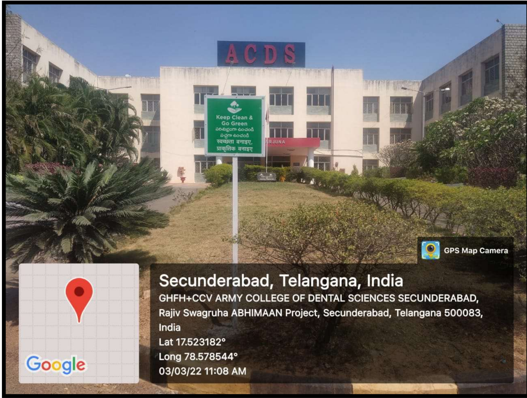
Fig-26: Signage- Keep clean and go green
