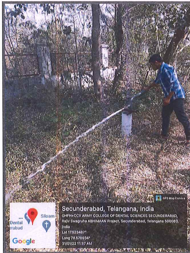
Fig-6: Bore well in the college campus
