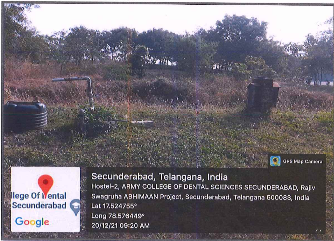
Fig-2: Bore well in the college campus
