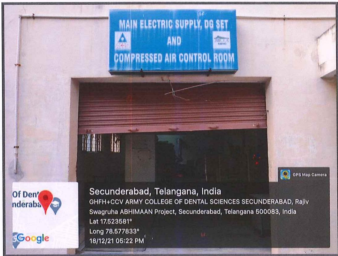
Fig-13: Main Electric Supply room
