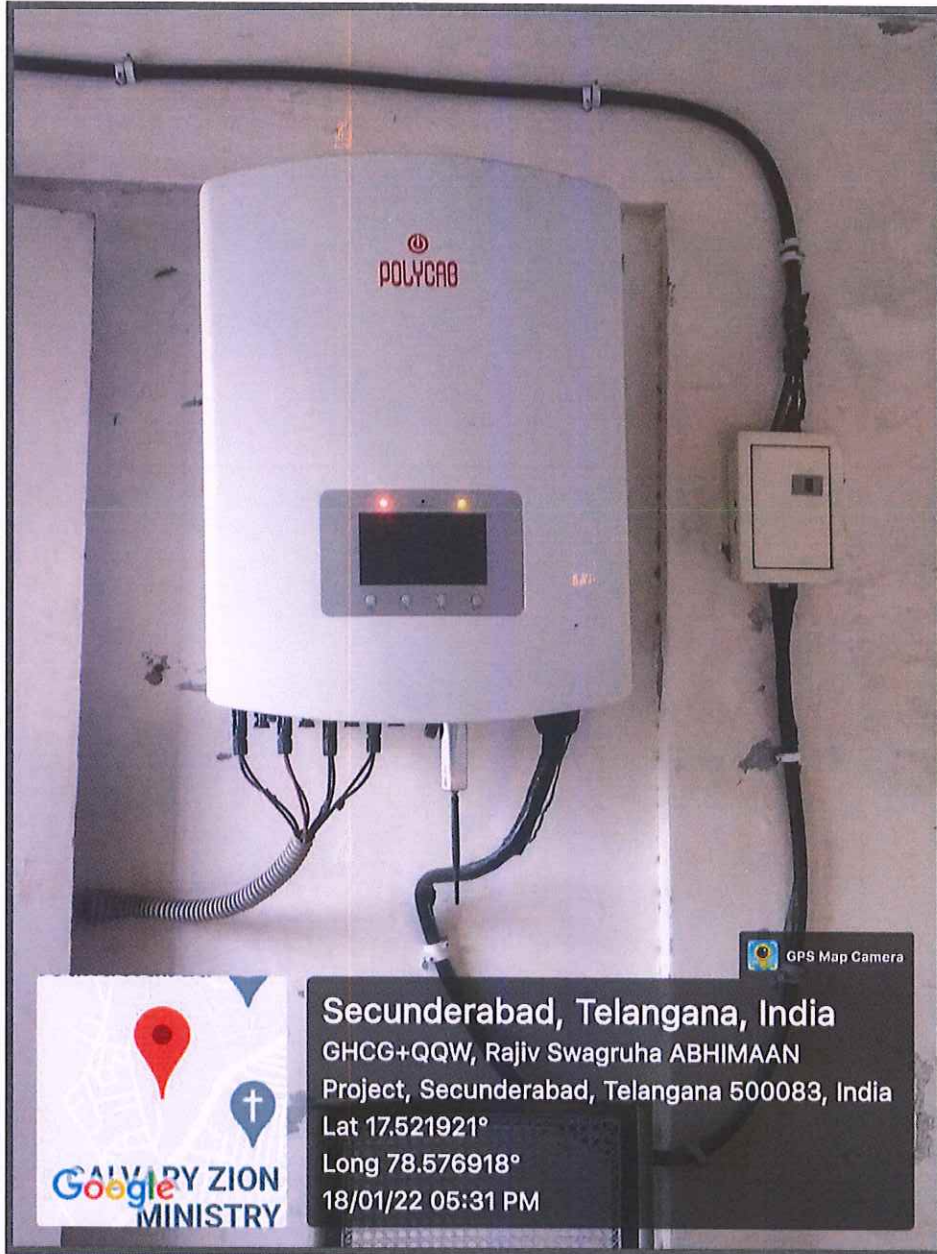
Fig-3: Polycab string grid tie inverter
